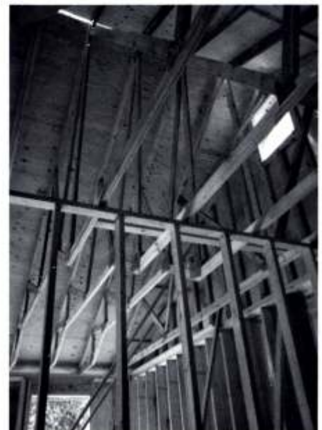
Figure 3. (Below Right) Partitions not near a truss joint, with a single top plate, and with studs between trusses, will not pick up much truss reaction.
